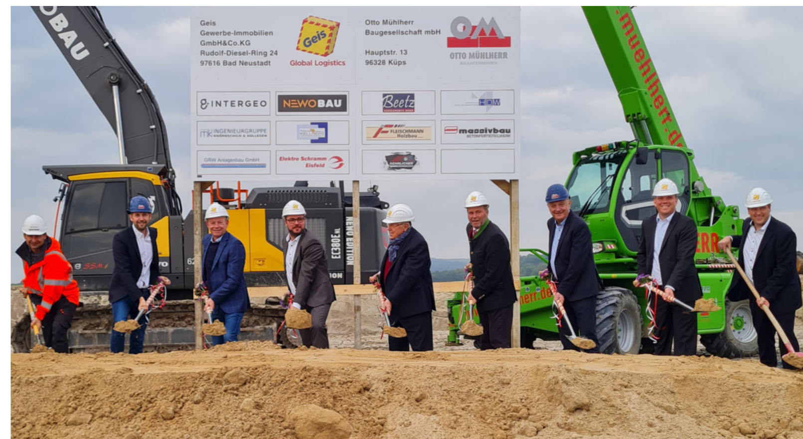
Groundbreaking in Ebersdorf in October 2022
